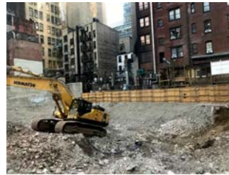
Excavation proceeding as of early May (CityRealty)
